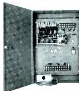
Typical Lamp Failure Indicator Panel
